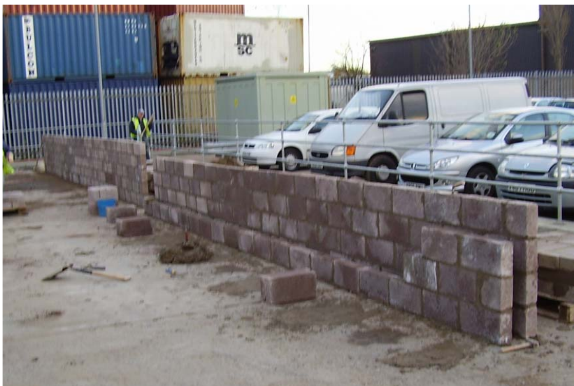
Figure 2: Walls built with Class 3 cement:lime:sand mortar
