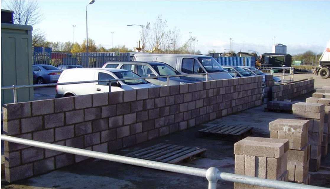
Figure 1: Walls built with Class 3 cement:sand mortar
